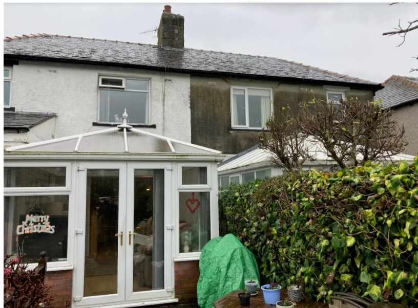
Photo 4: Rear of no. 265 (left) and Rear of no. 267 (right)
