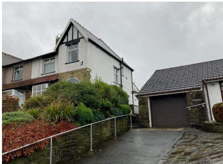
Photo 2: Side of no. 265 (left) and as seen from driveway of 261 (right)
