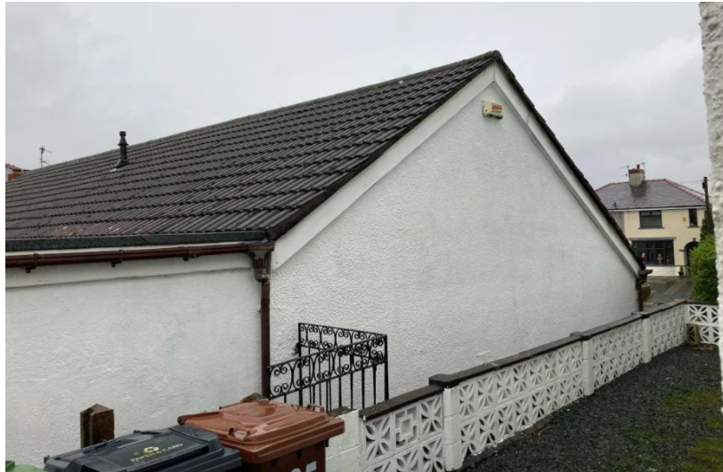
Photo 6: Showing relationship with neighbouring property. Side elevation of no. 261 and side yard of no. 265.
